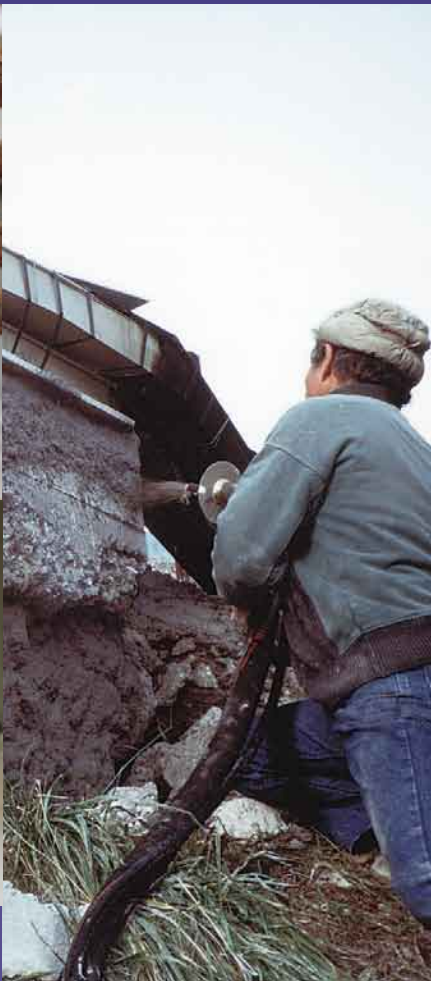
Remove spalled concrete from deteriorating structure.
